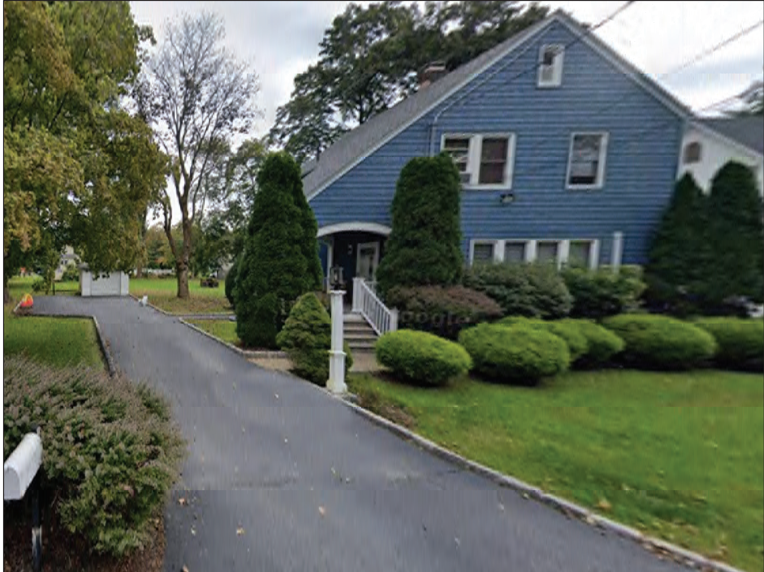
FRONT VIEW OF EXISTING HOUSE - LOT B
